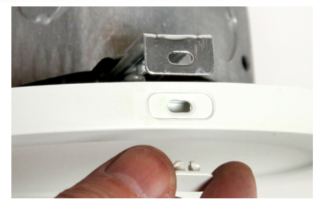
Put light onto crossbar and install tab
