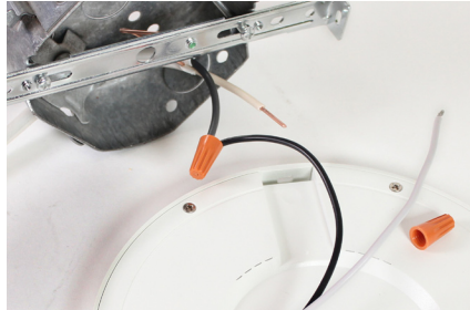
Connect wires with wire nuts / marettes
